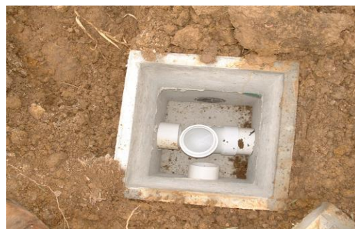
Figure 20. A 90° elbow used as a flow diverter.
