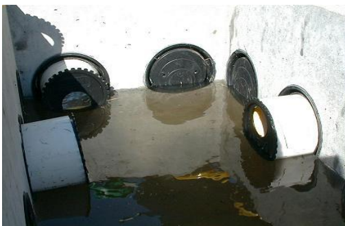
Figure 19. Speed levelers installed on both outlets as flow diverter.
