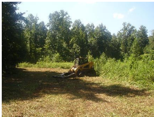
Figure 2. Area being cleared of high weeds with a bush hog in preparation for system installation.
