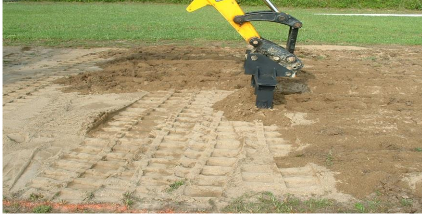
Figure 15. Shows a thin sand layer being plowed into soil surface (method #2). Note: equipment was driven perpendicular to length of mound (see tracks).
