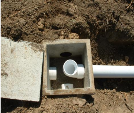
Figure 18. A 4-hole distribution box with plug (one knockout not removed) is used as a diversion device.
